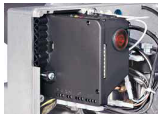
Control box fitted with ignition transformer
